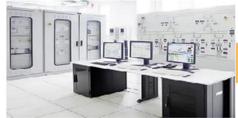
We are expert in manufacturing DG synchronizing system which are used for automatic changeover from E.B mains to DGs at the time of E.B failure. When the E.B mains supply is restored, the system automatically changes back and stops the DGs.
